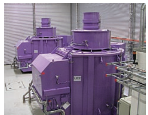
A special colour for special machines: the first hydro-electric generators that LDW supplied to Greenland are in Sisimiut.
